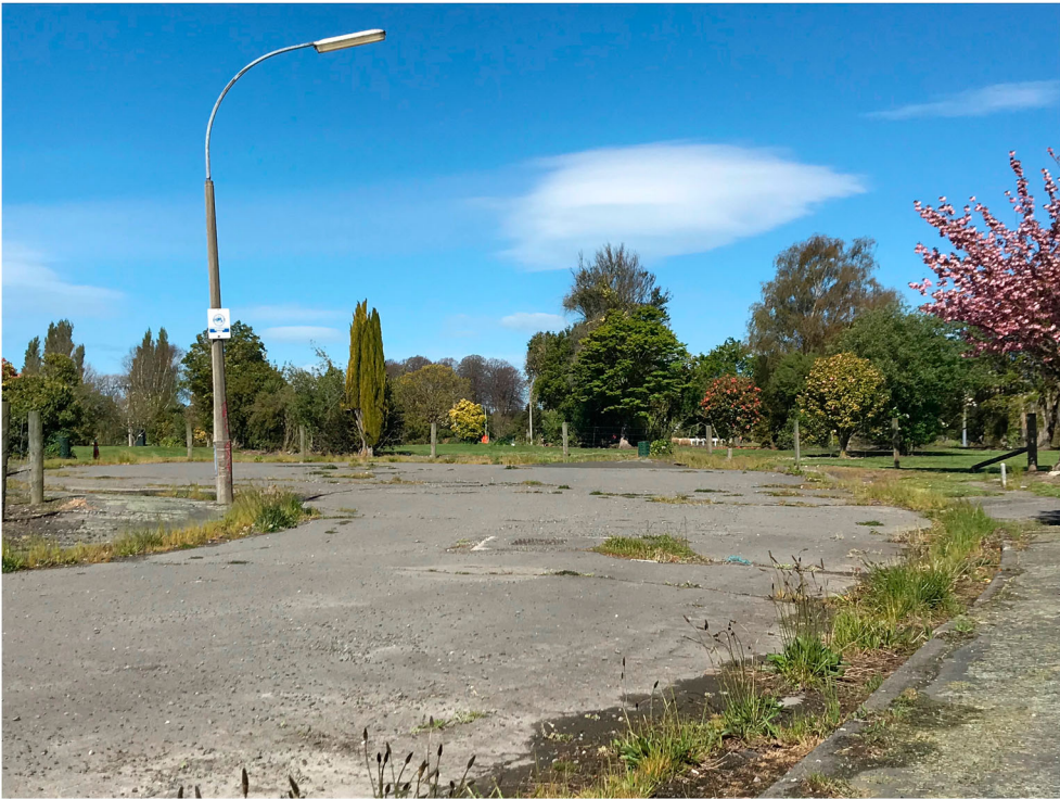
Figure 3. Abandoned red zoned street in Avonside, October 2018. Photograph: Eric Pawson.
